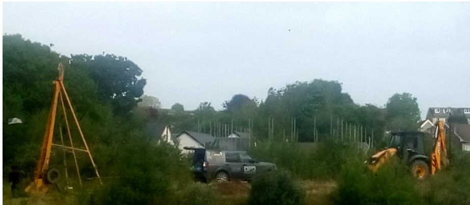
Site investigations for foundations.
